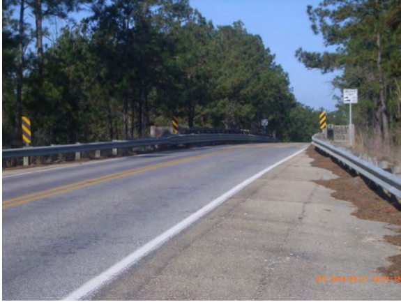
LA 36 looking westbound at RR Overpass
