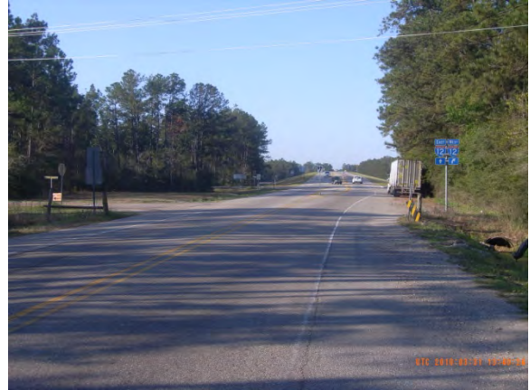
LA 434 looking southbound at I-12
