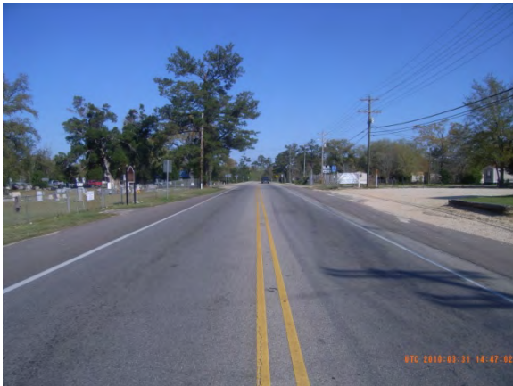
LA 41 looking northbound near LA 36 intersection
