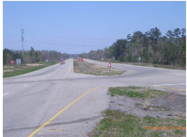
LA 41 looking northbound at LA 21 Intersection
