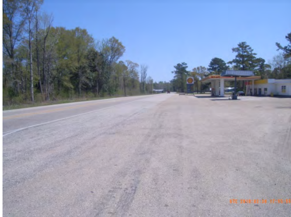
LA 21 looking eastbound at LA 40 Intersection
