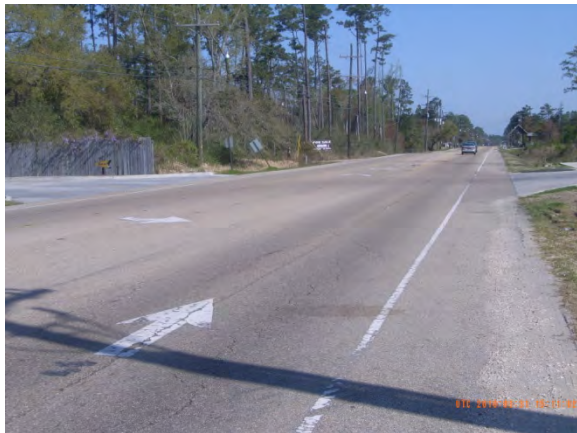
LA 21 looking southbound near Bush
