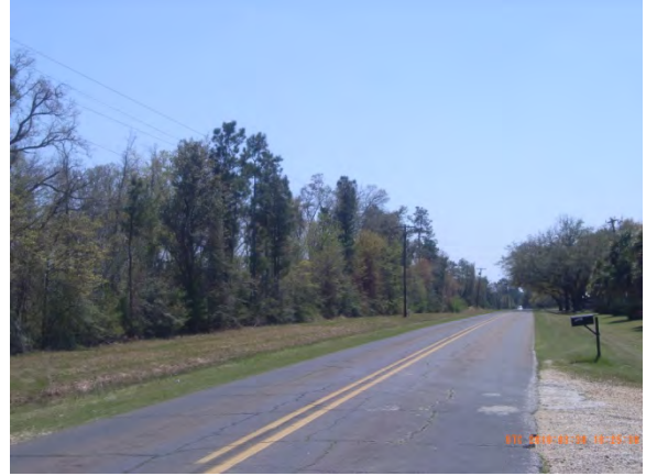
LA 1083(Allen Rd) looking northbound near Sanders Road
