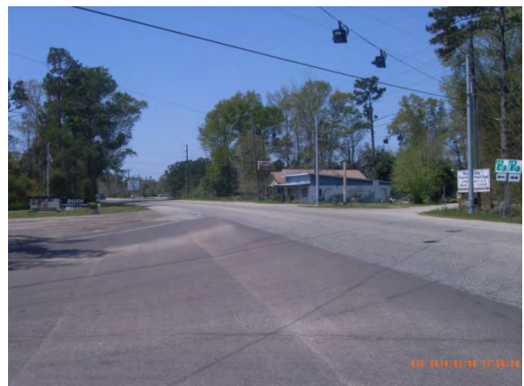
LA 21 looking westbound at LA 40 Intersection
