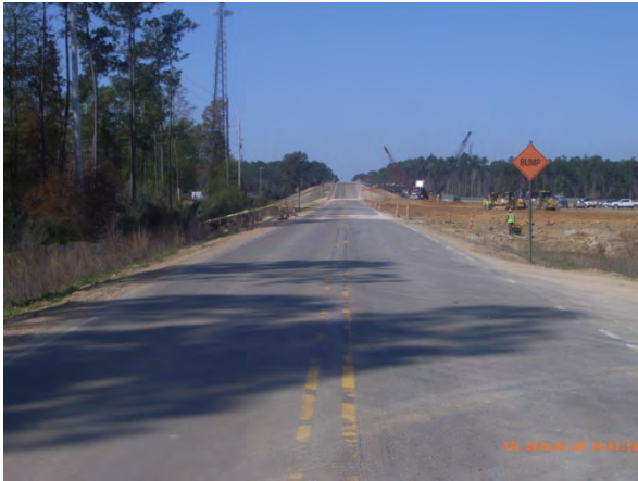
LA 1088 Looking southbound toward I-12 (Construction of LA 1088 Interchange in Progress)
